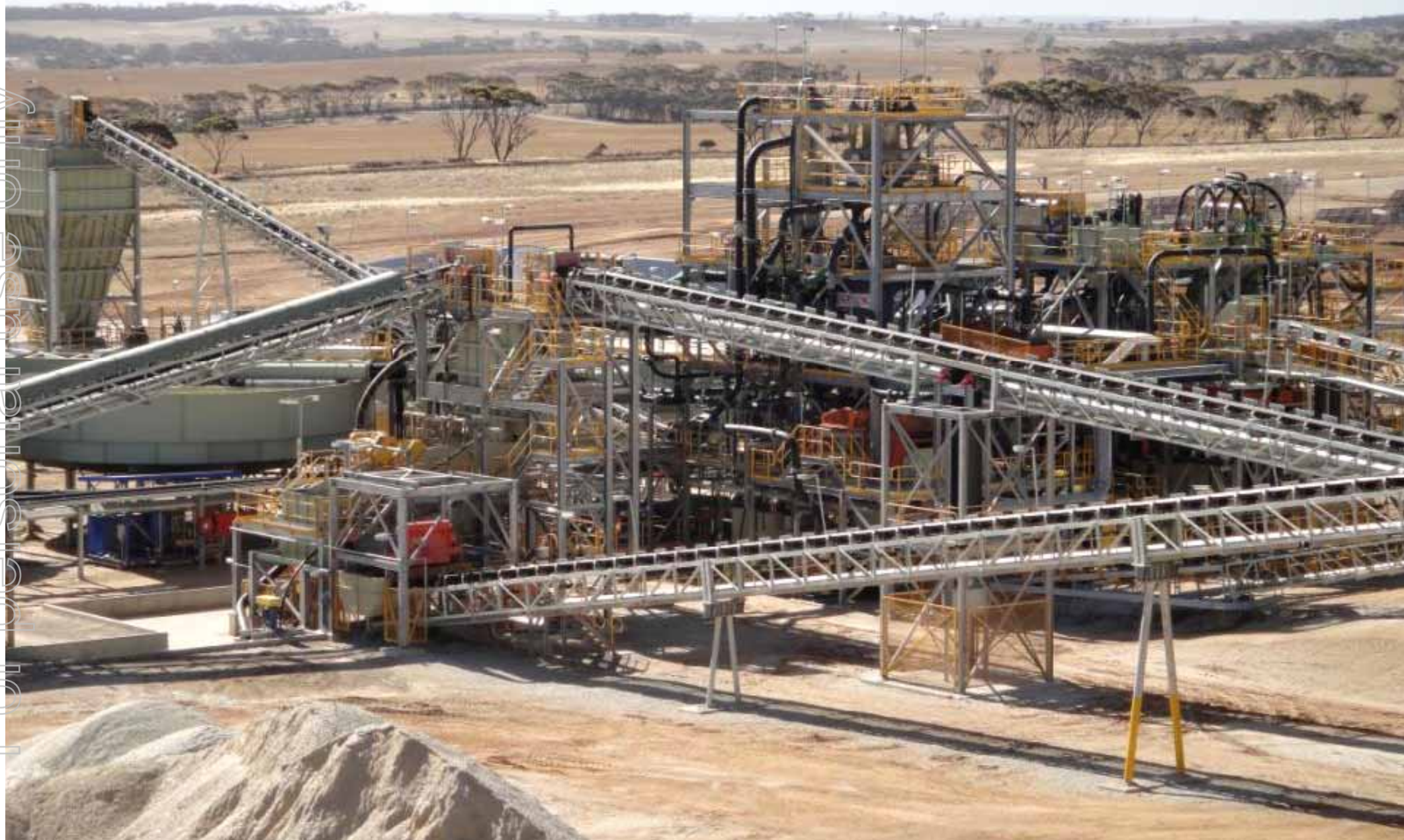
Primary screening plant
