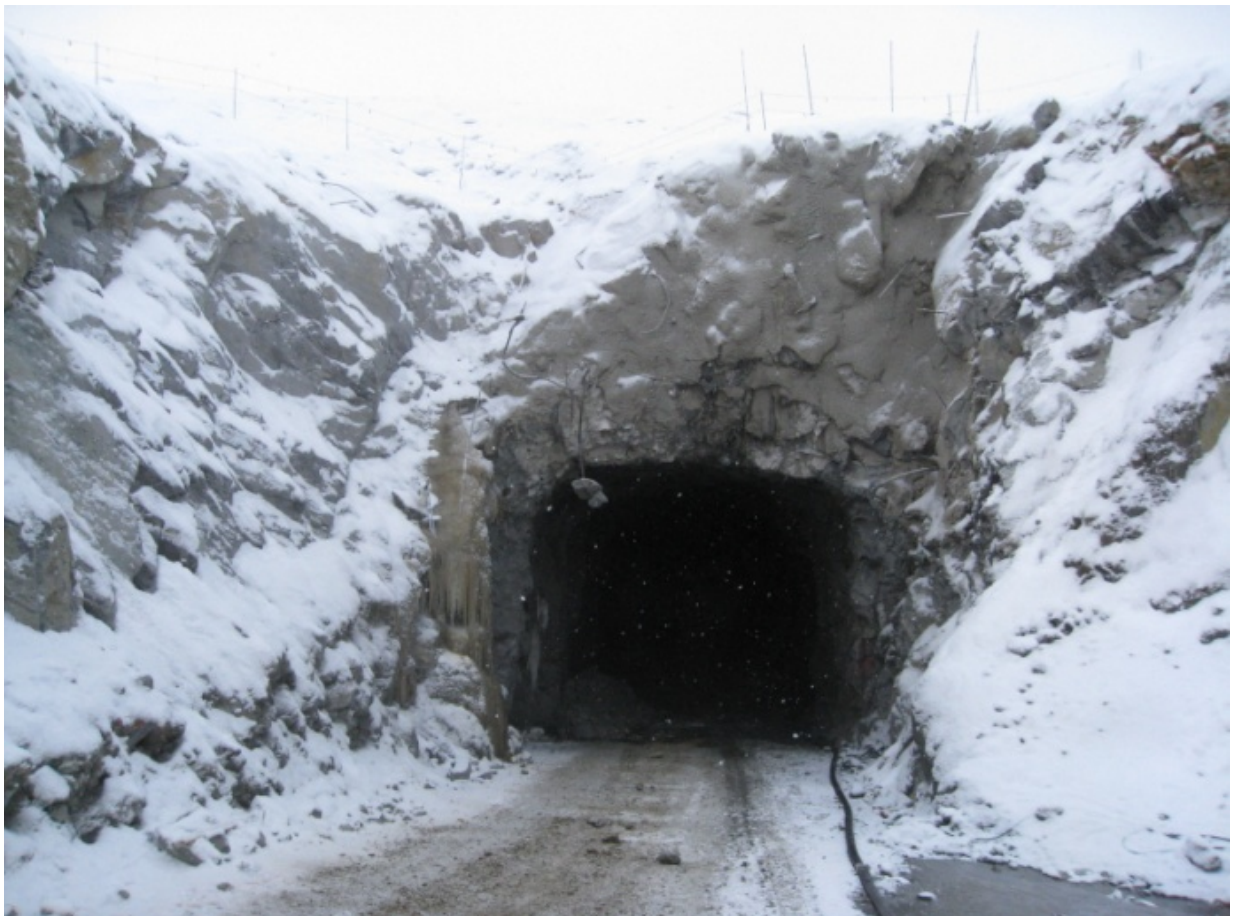
Kylylahti mine portal
