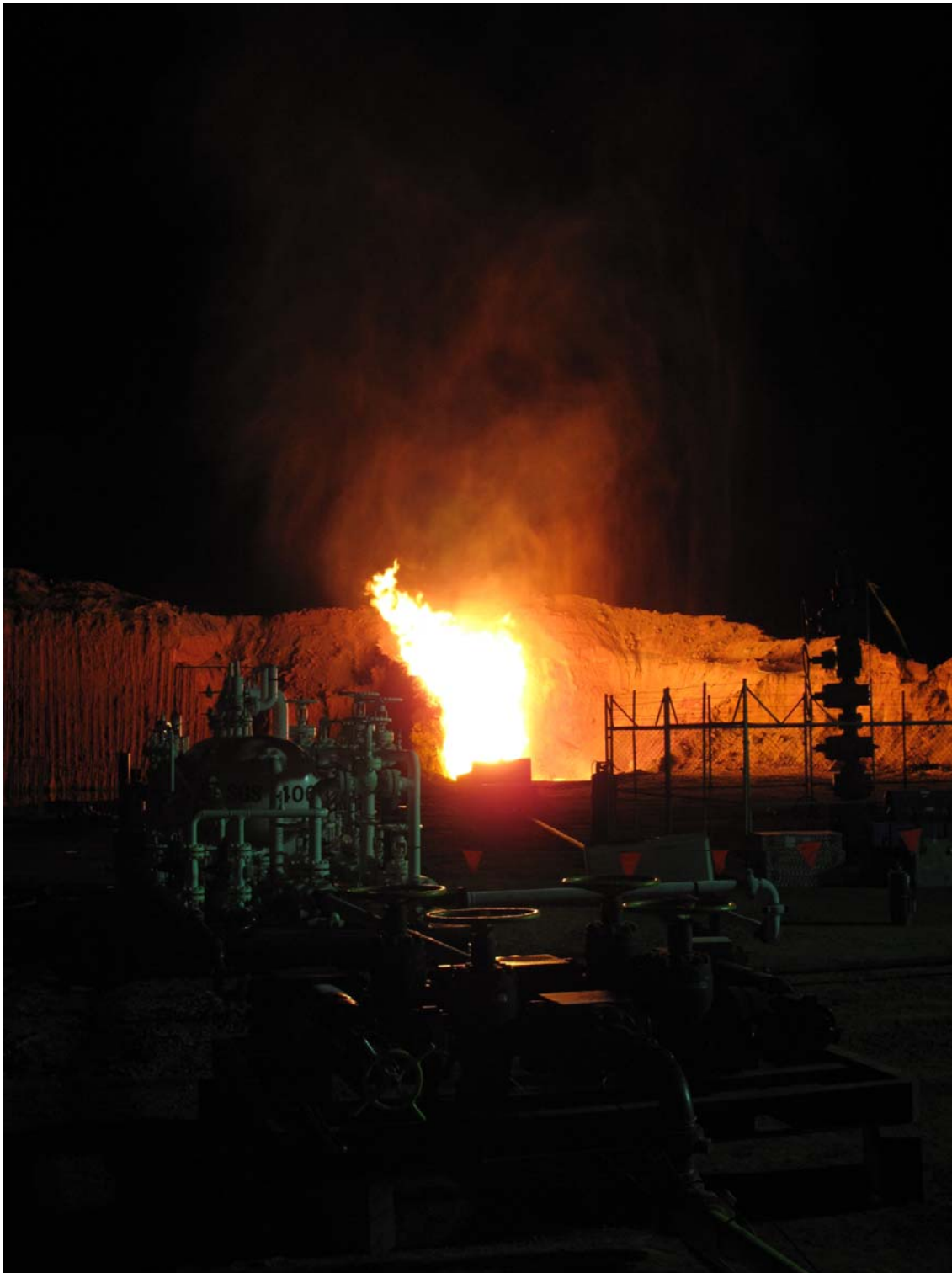
Red Gully-1 flowing Gas and Condensate. SGS Gas Separator in foreground. The Gingin West-1 well, drilled in November 2009 and Production Tested in July 2010, on the right. Flare pit in the background.
