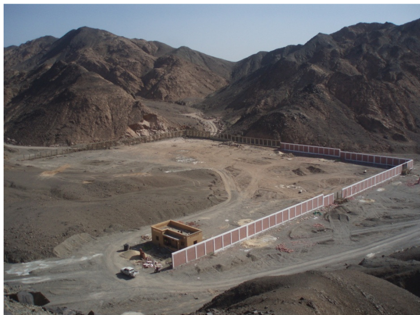
Figure 1: Construction Progress as at 5 April 2011
