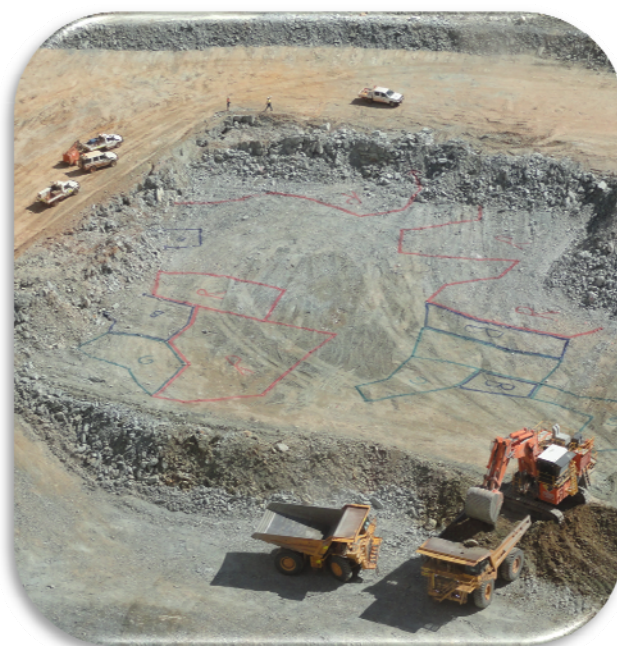
Photo 2: Excavator in Central Pit – April 2011
