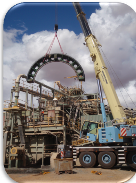
Photo 3: Mill shutdown work – February 2011
