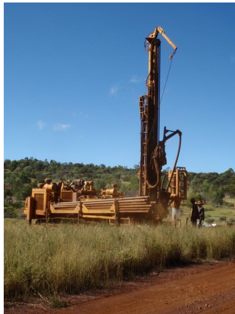
Drilling Greenvale Resources
