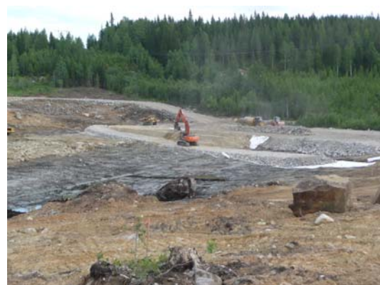
Earthworks at concentrate storage dam
