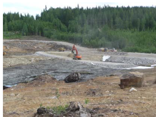
Earthworks at concentrate storage dam
