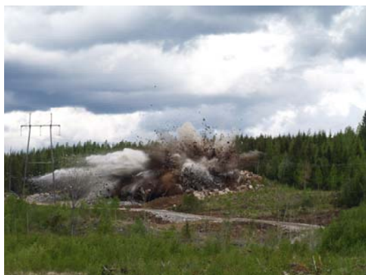
Blasting for site preparation at concentrate storage dam
