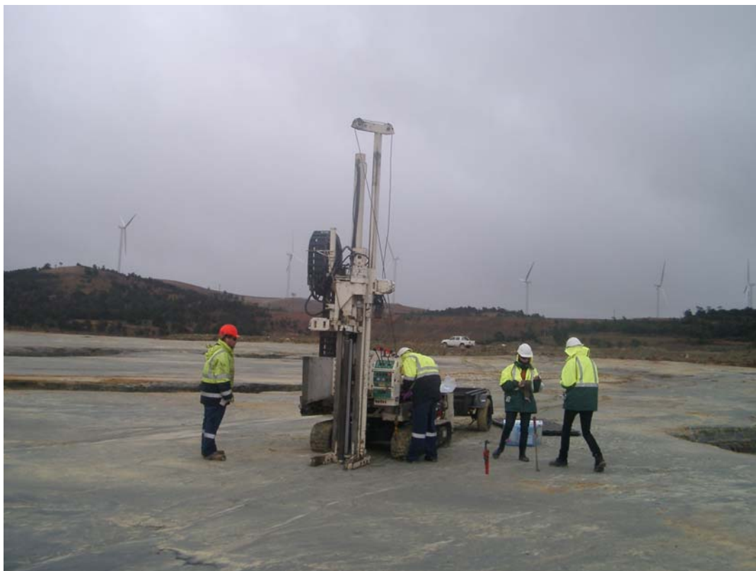
Figure 1: Drilling on Tailing Dam South, the Woodlawn Retreatment Project.
