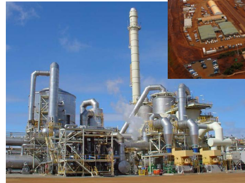
BHP's acid plant at Ravensthorpe, WA (below)
