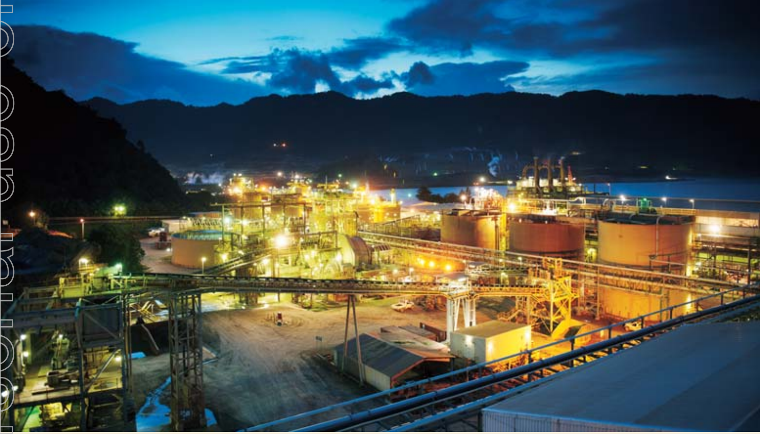
Above/ Lihir processing plant at night
