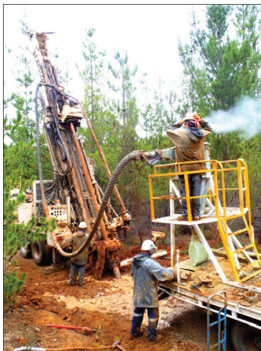
Figure 4 – Reverse Circulation Drilling at the Barnes Hill Project, Tasmania
