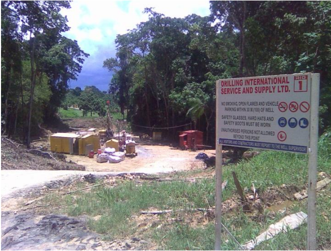
Figure 4 – Rig 1 on Location in Trinidad
