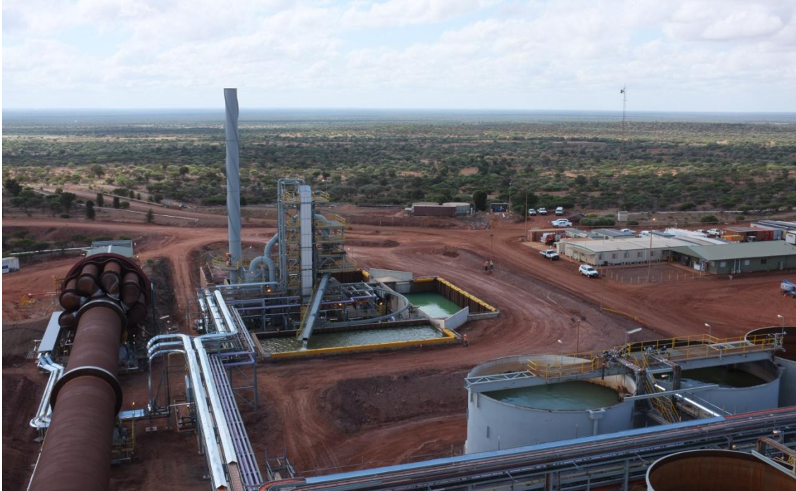
Kiln and leach vats undergoing wet commissioning
