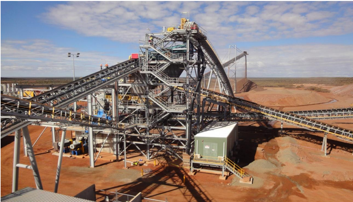
Building of the crushed ore stockpile
