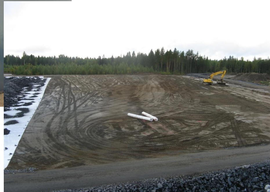
Installing the lined base of the ROM pad
