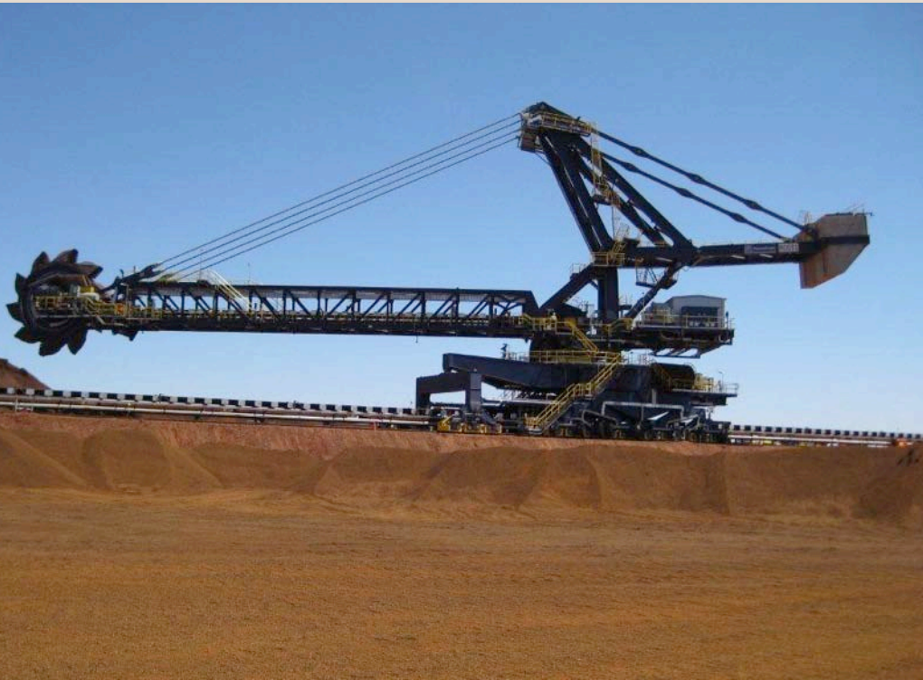
Christmas Creek ore load-out reclaimer, October 2011
