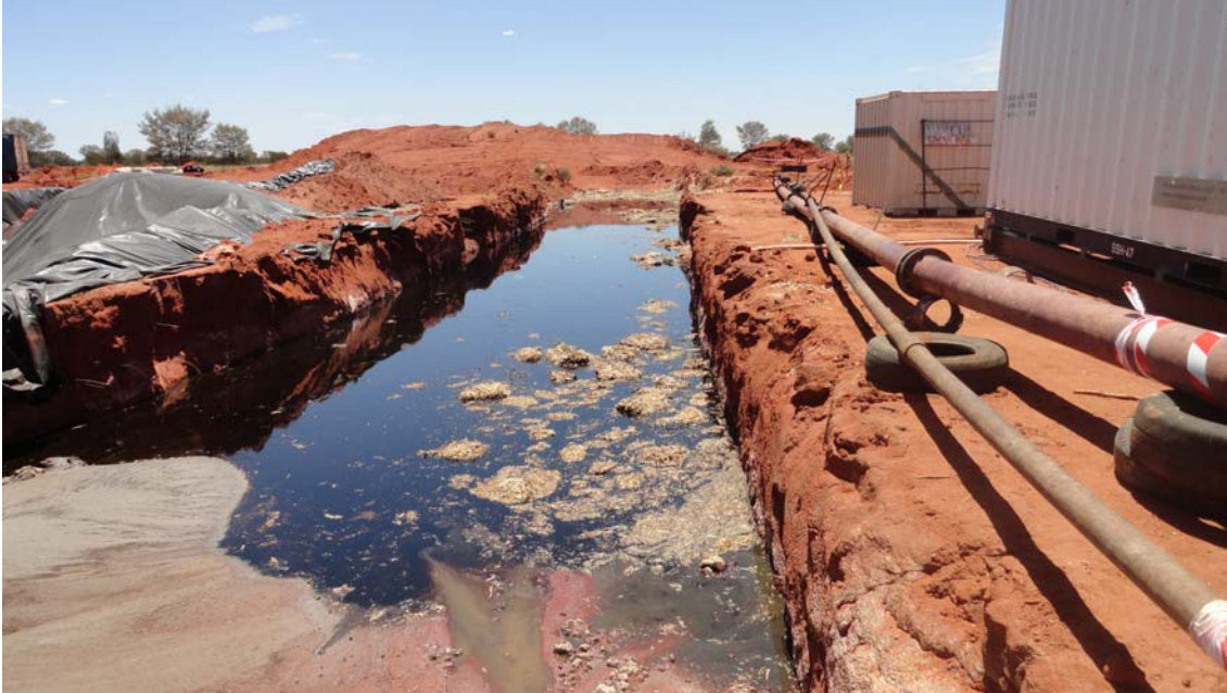
Layer of oil on surface of sump during drilling. This has now been skimmed off and stored in environmentally safe containers for later disposal.
