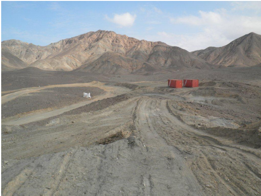
Figure 4: Pre-production earthworks at the ore processing site
