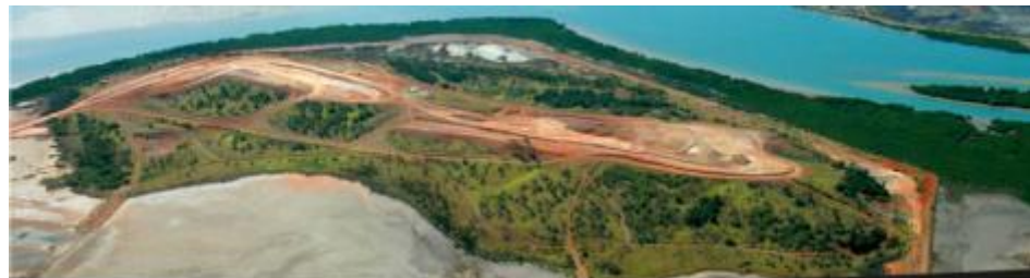
Wiggins Island Coal Terminal site location, September 2011 Source: www.wicet.com.au website
