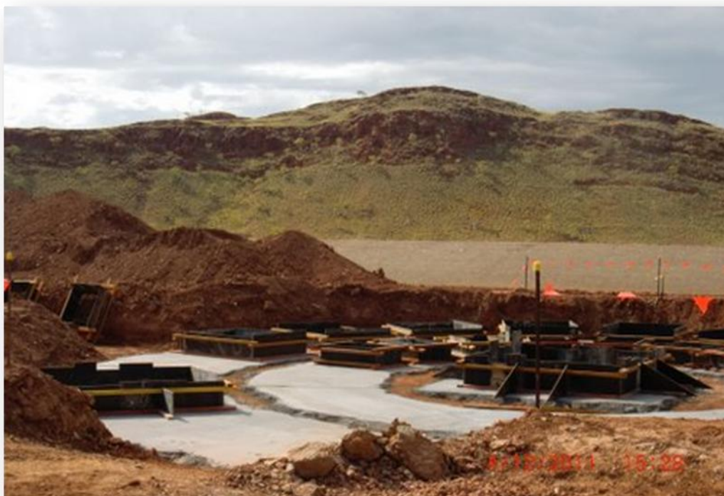
Form work positioning for thickener
