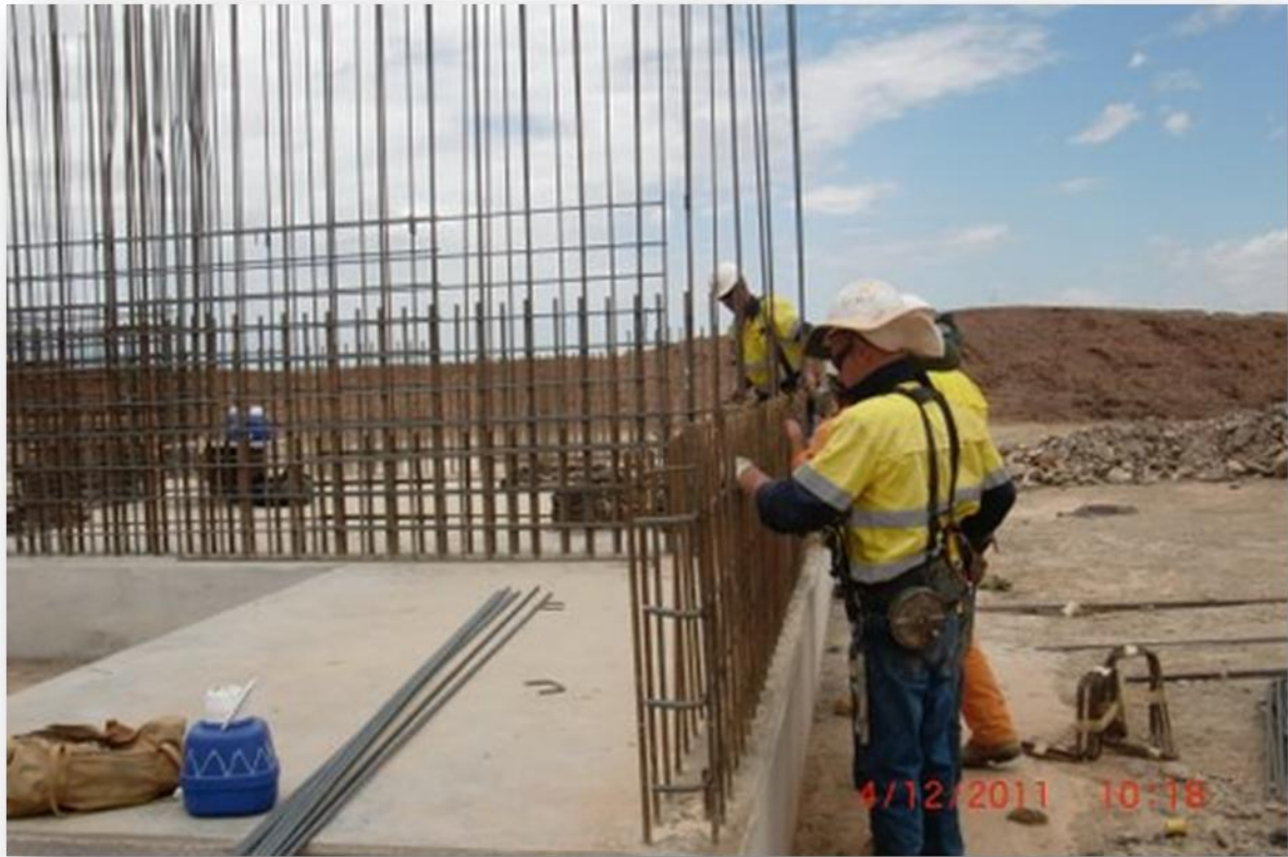
Crusher Wall rebar
