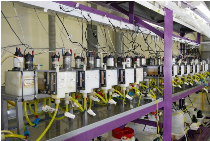
Solvent Extraction Circuit for REO Production 2012 ANSTO, Sydney
