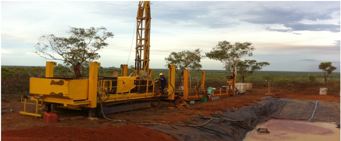
Figure 2 – Drilling of the first 110m of LBD03 at Lindeman’s Bore
