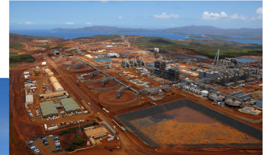
Goro nickel plant in New Caledonia (above)
