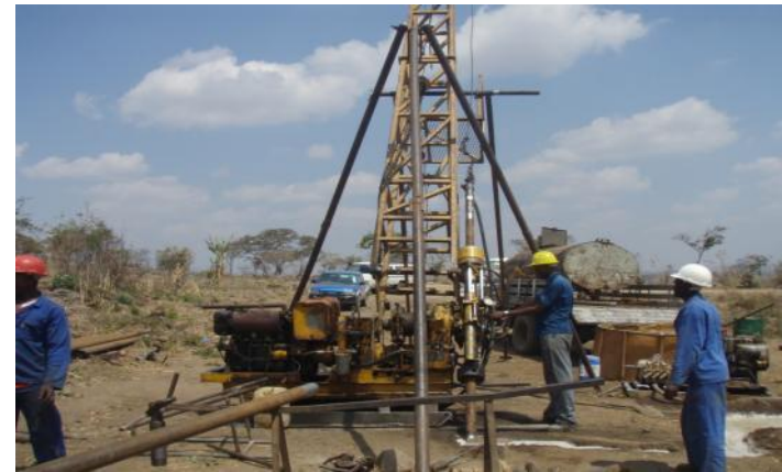
Drilling at Kanyika
