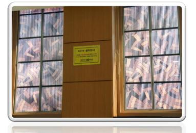
Dye Solar Cell technology is a biomimetic nanotechnology that emulates the natural process of photosynthesis. Using a layer of titania, electrolyte and ruthenium dye sandwiched between glass, DSC technology generates electricity when light striking the dye activates electrons which are absorbed by the titania to become an electric current.
