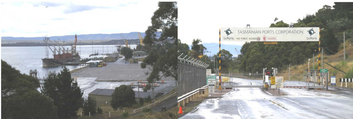
Figure 2 – Deep-water Port at Bell Bay
