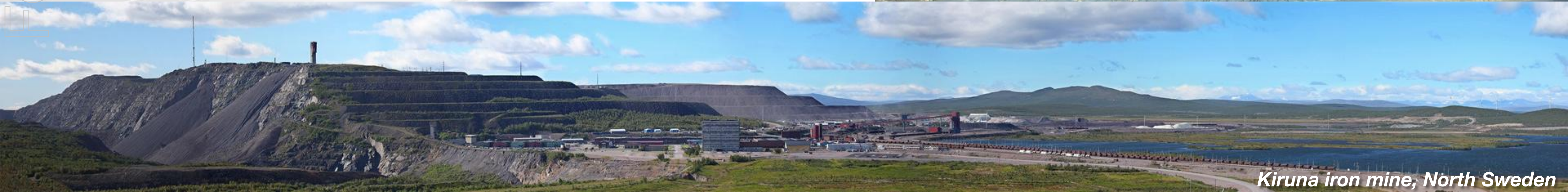
Grid power near projects
