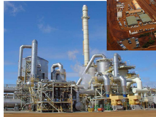
Acid plant at Ravensthorpe, WA (below)
