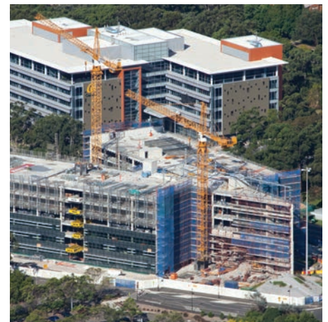
Construction progress at Macquarie University's Australian Hearing Hub
