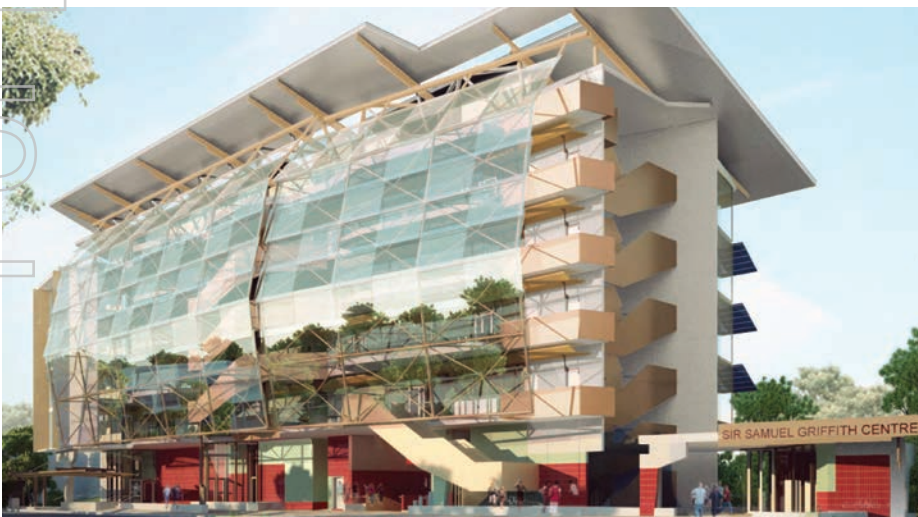
Sir Samuel Griffith Centre – Australia's first zero-emission, self-powered education building driven by solar-hydrogen energy. (Image courtesy of Cox Rayner.)
