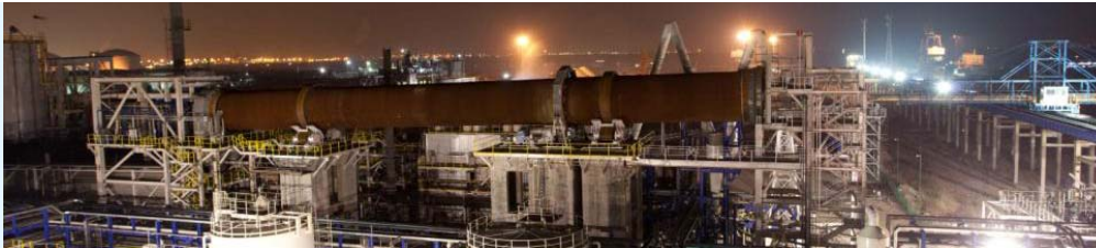
Jiangsu LC Plant (China)
