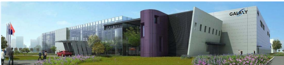
Jiangsu Battery Project (China)
