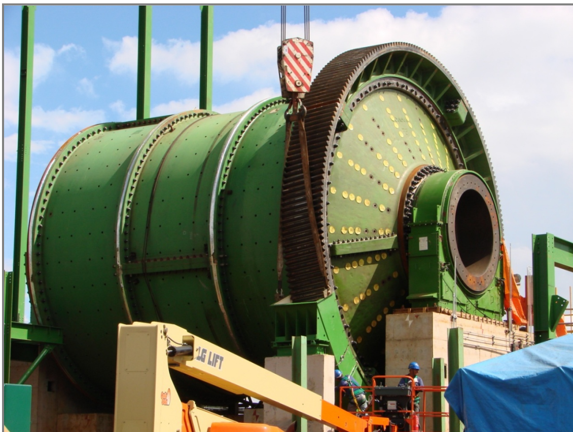
Photo 4. SAG Mill 75% complete (note tradesmen in foreground for scale)
