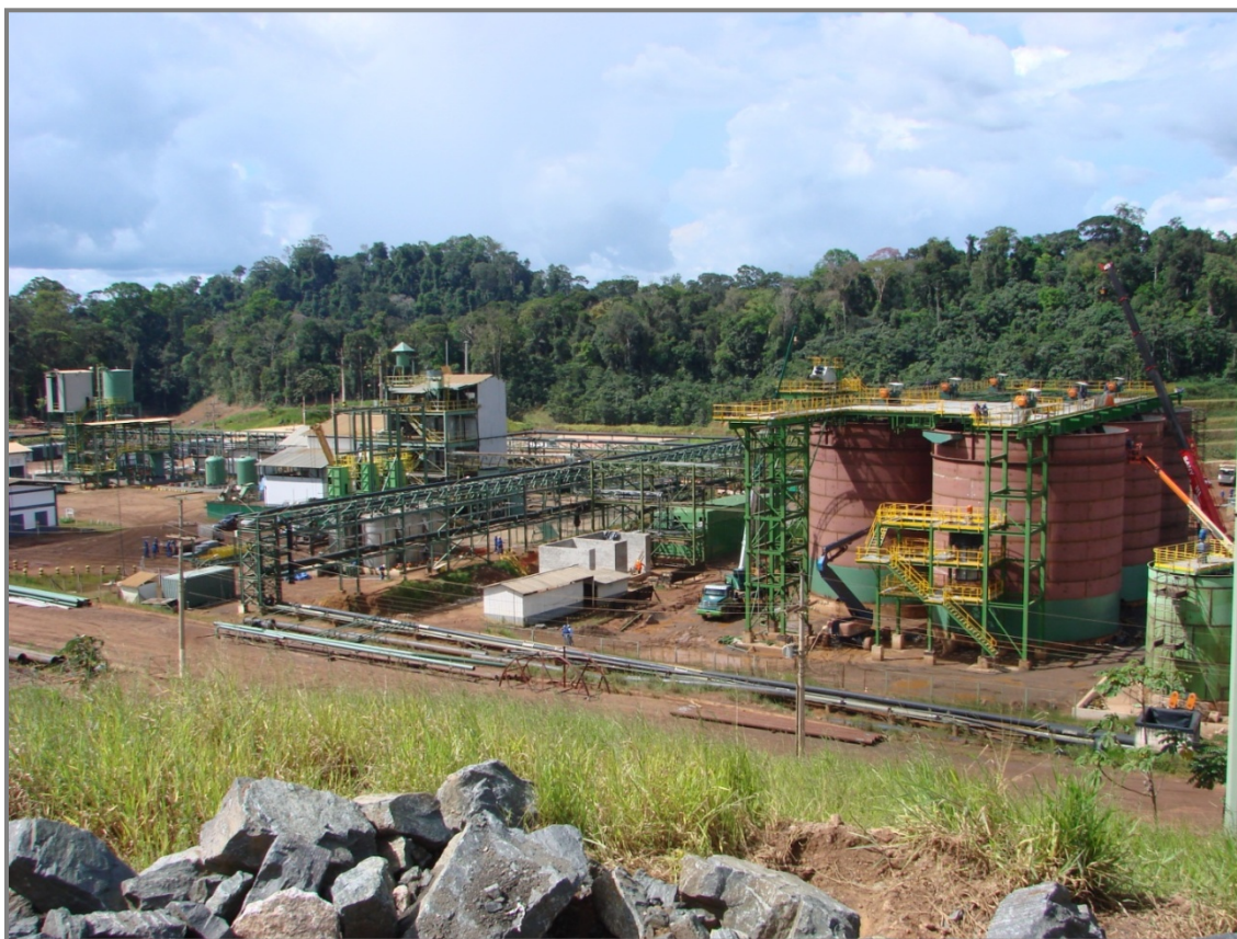
Photo 1. CIL Tanks and Gold Elution Circuit
