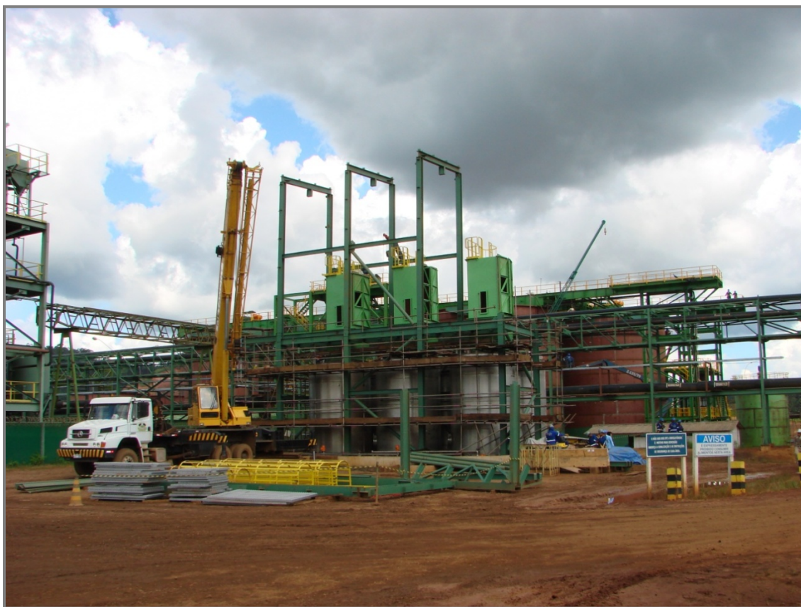
Photo 3. Reagent area with CIL Tanks in the background
