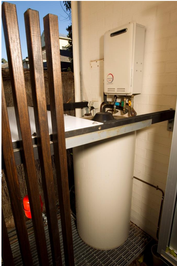
200 litre hot water tank & booster
