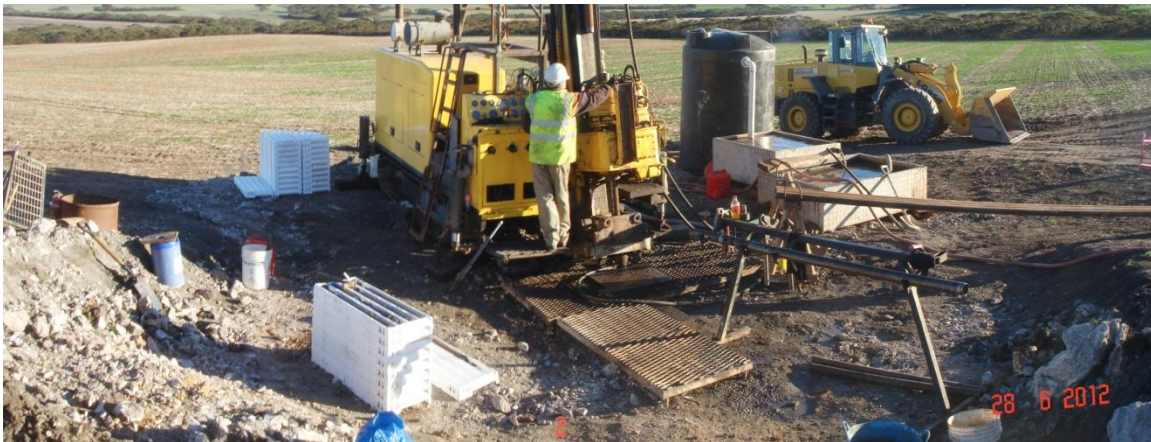
Plate 2. Photo showing diamond drilling in progress for hole CSDD12_003
