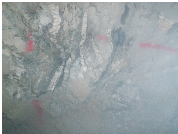
Sublevel 3 south 6 face at end of the period.
