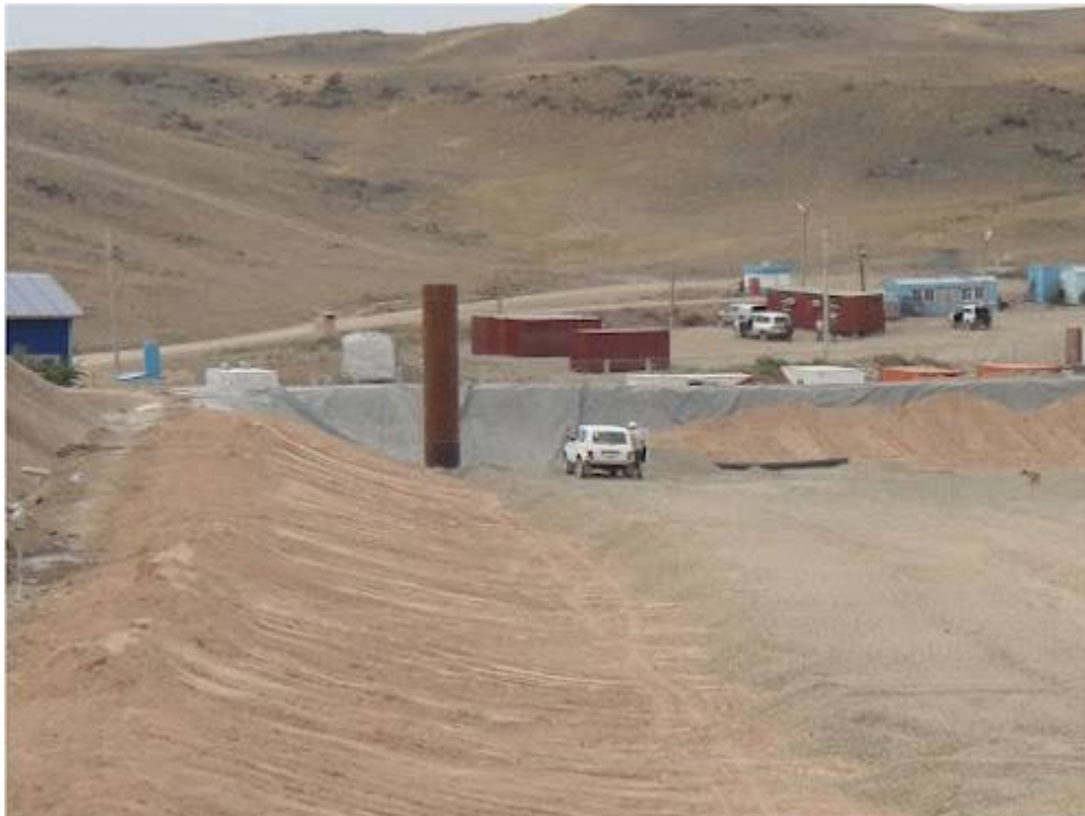
Heap leach pad number 2 at the Dalabai Gold Project, Kazakhstan
