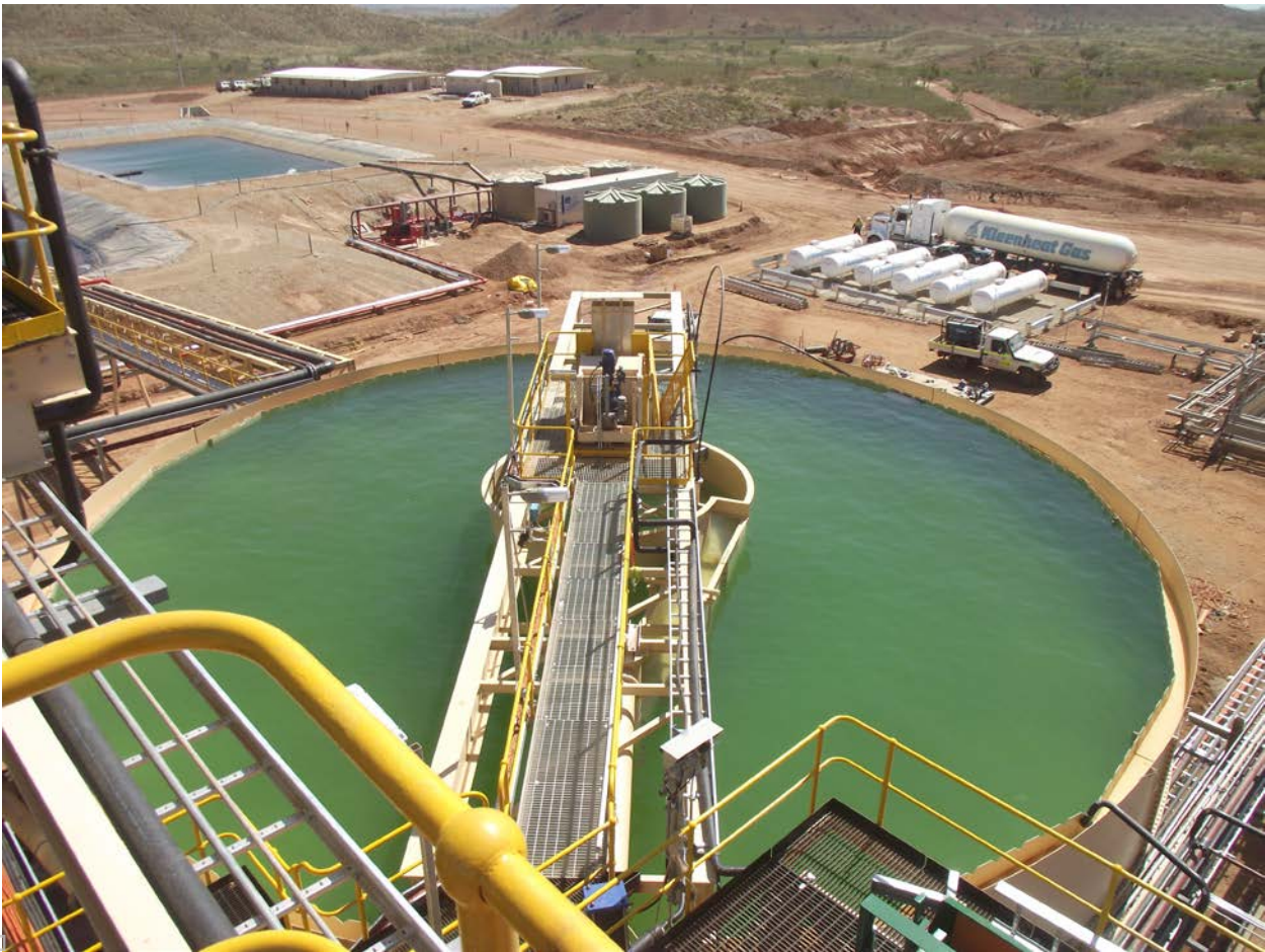
Hydrostatic Testing of the Tailings Thickener
