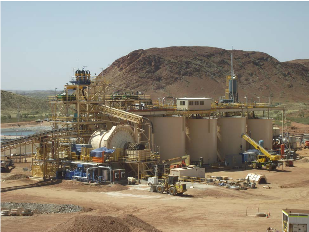
Nullagine Process Facility – Final Clean Up
