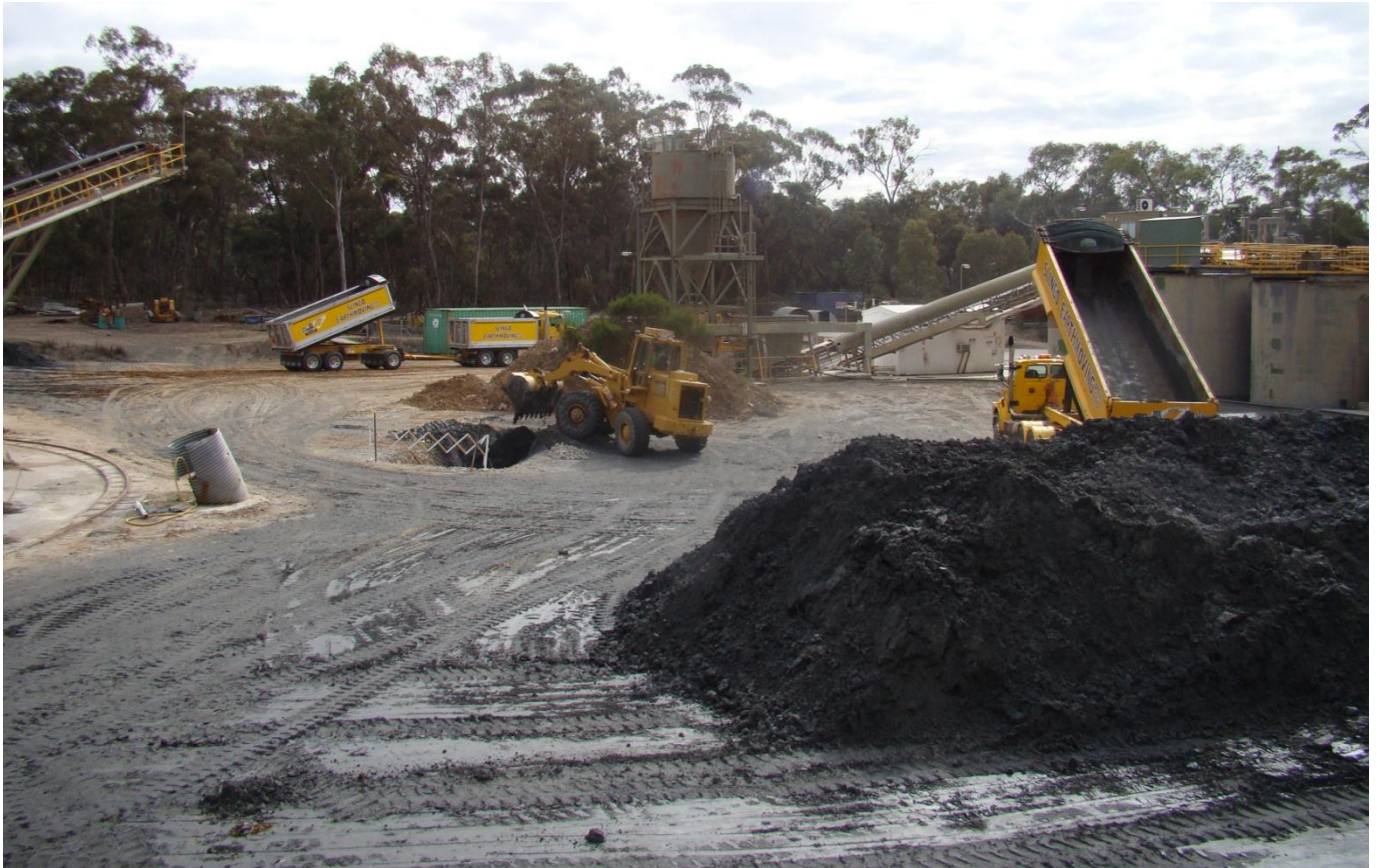
Tailings delivered to the Porcupine Flat Gold Processing Plant with loader feeding the ore shoot
