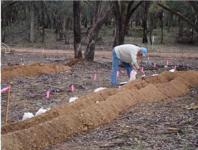
Surface trenching and grade control sampling
