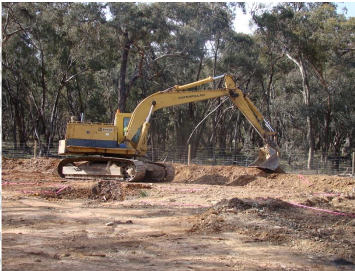
Construction of open pit bund wall
