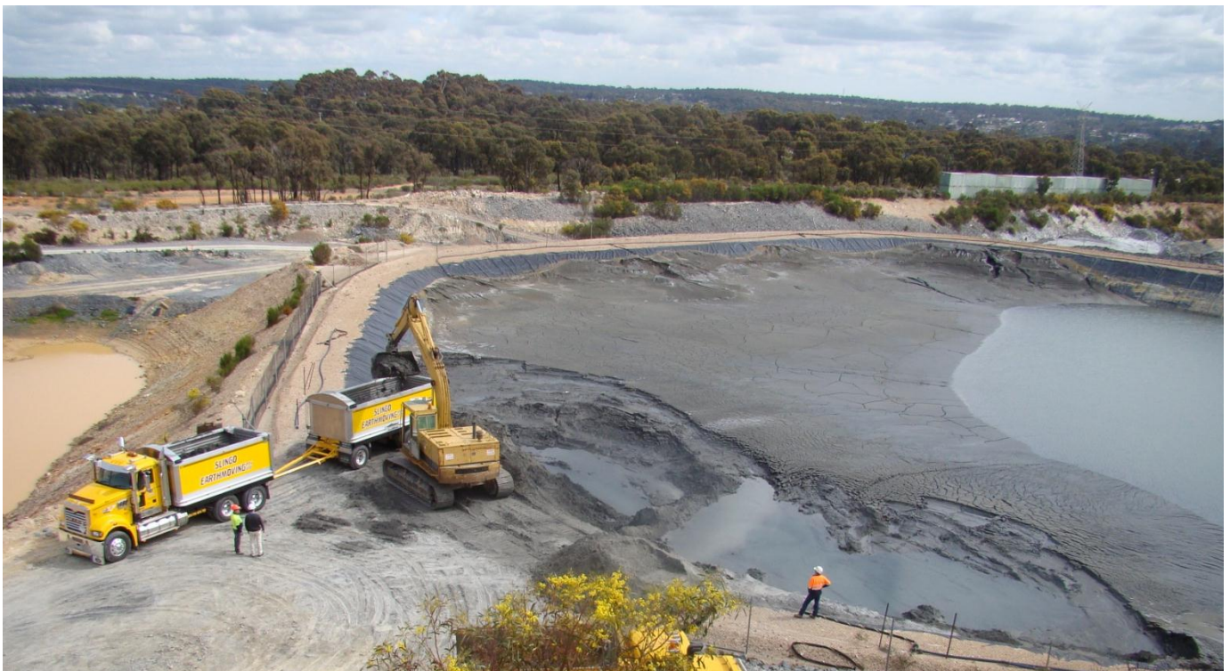
Excavator removing tailings from the flotation concentrate tailings dam at the Kangaroo Flat Gold Mine
