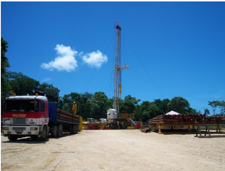
Figure 3 – Drilling Rig on Location
