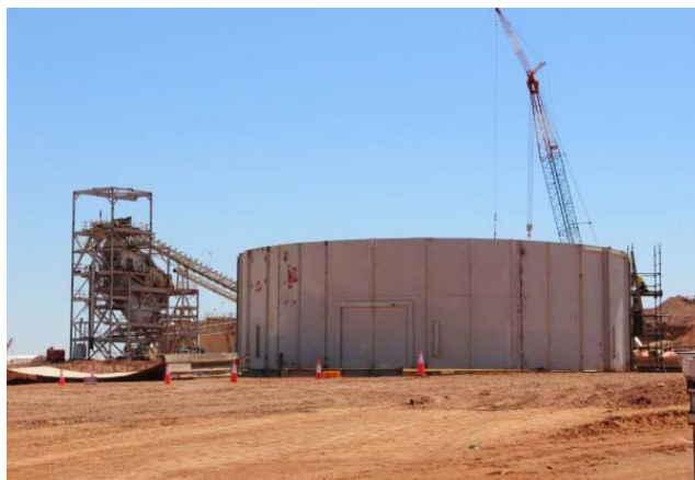
Fine Ore Bin Construction
