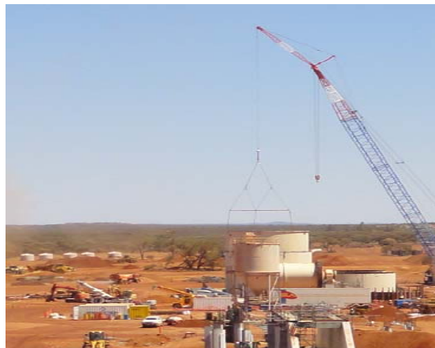
CIL Tank Construction
