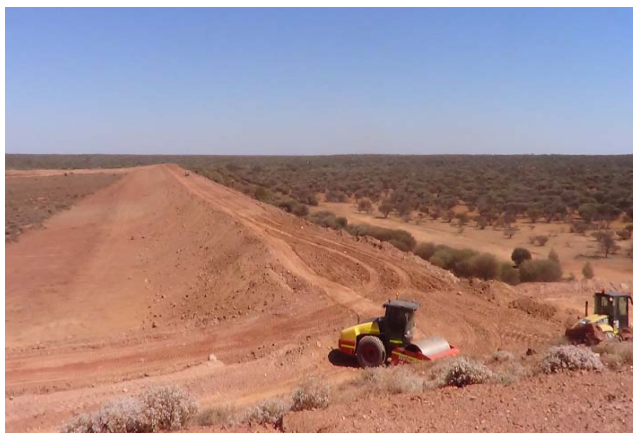
Tailings Dam Lift Under Construction
