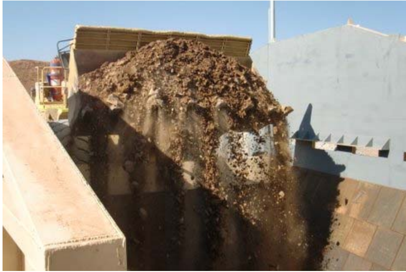
First Rock to Crusher 26 August 2012 & stockpile establishment
