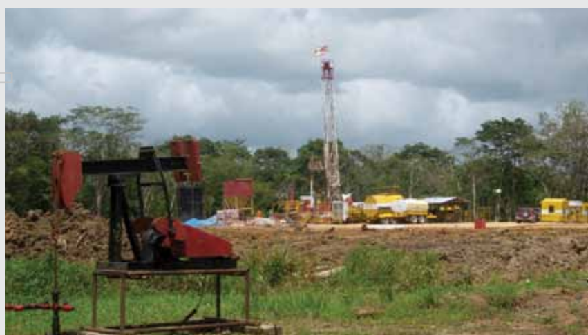
Figure 4 – Drilling Rig on Location
