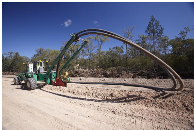
Iplex pipe being installed Queensland, Australia
