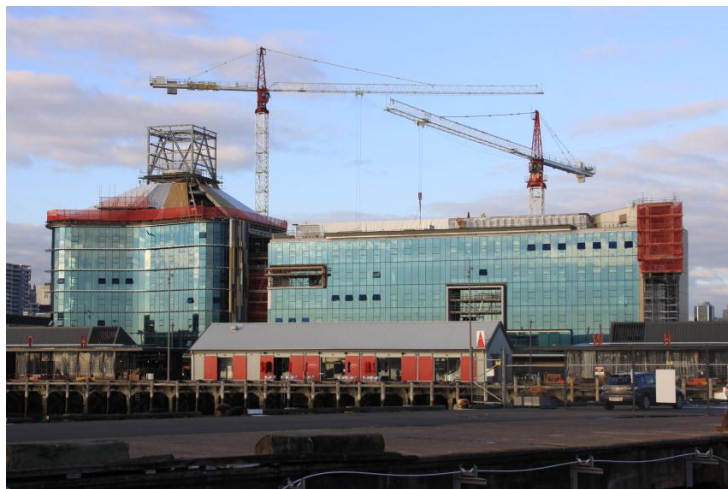
ASB North Wharf Auckland, New Zealand
