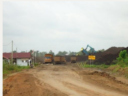
Jetty access road
