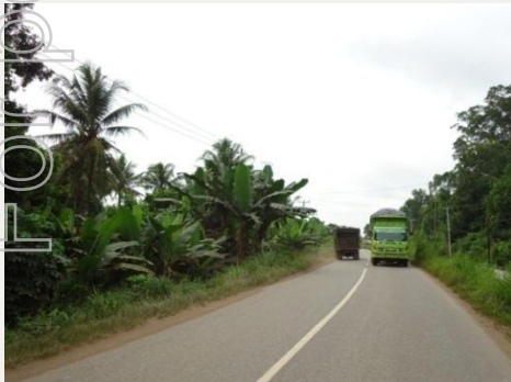
Sealed Haul road
