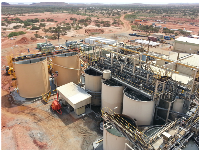
Figures 3 - New leaching tanks and Knelson Concentrator
