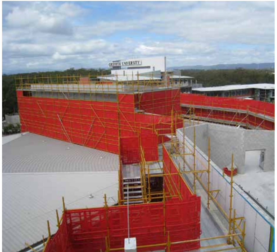
Works are progressing well on the Griffith University project
