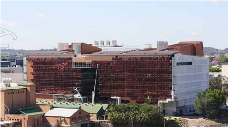
The first stage of the Translational Research Institute was completed on time and handed over to the client in November 2012. Photo courtesy of the Translational Research Institute (Wilson Architects and Donovan Hill)
