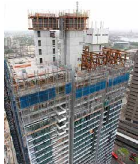
Construction progress on One Central Park's east tower
