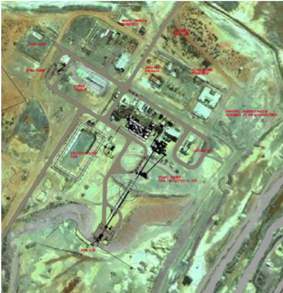
Figure 6: Plan of the CMGP mine site showing the processing plant and associated infrastructure
