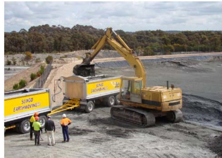
Excavator removing tailings from Kangaroo Flat tailings dam
