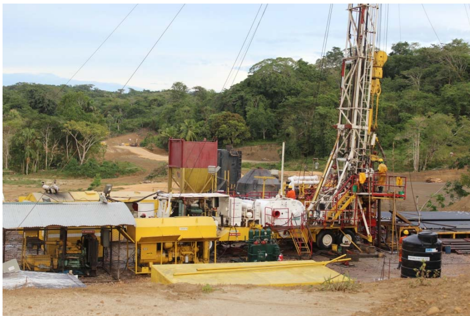
Figure 1: QUN 135 well drilling
