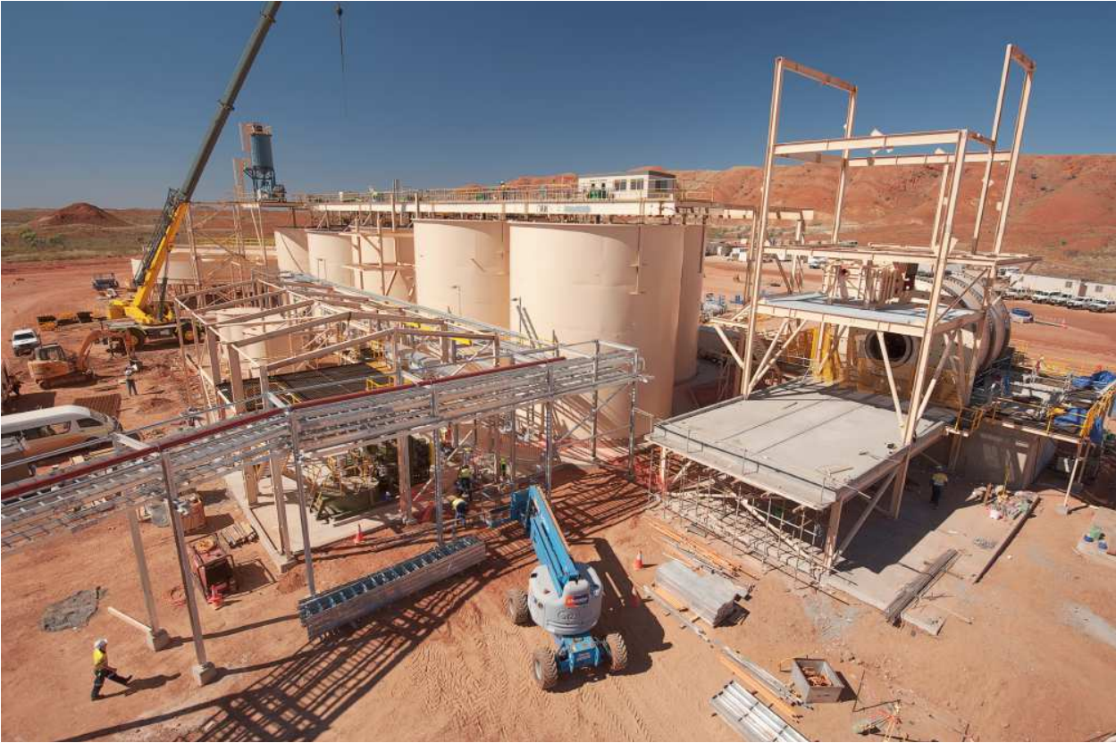
June 2012 – Mill Installation (right) and Gold Room Construction (left)
