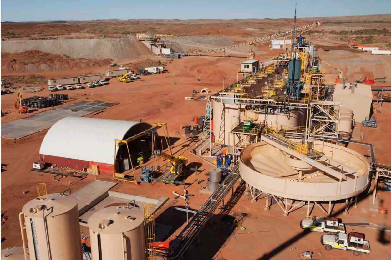
August 2012 – Process Plant Largely Complete. Thickener in foreground
