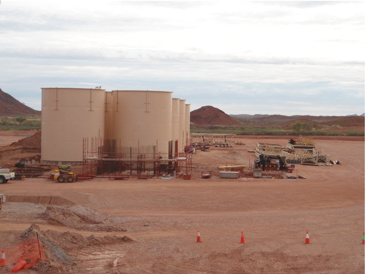
February 2012 - CIL Tank Installation
