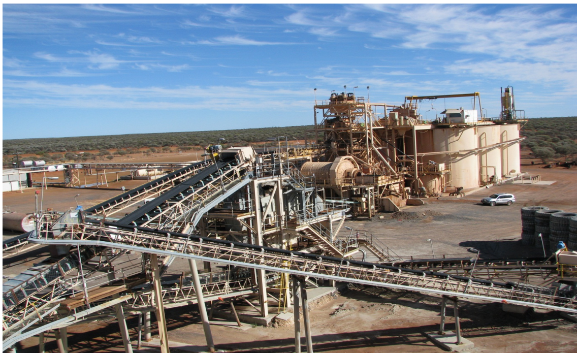
Figure 1: Existing Kirkalocka Processing Plant
